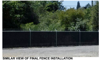
SIMILAR VIEW OF FINAL FENCE INSTALLATION
