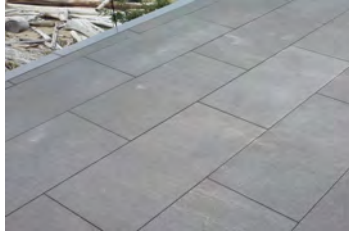
Balsalt Feature Paving
