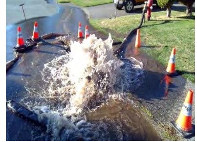
Typical set-up for water hydrant flushing.
