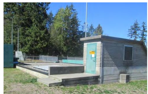
Newton Pump Station Sept 13, 2016
