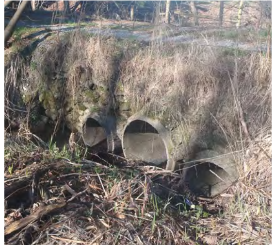
Existing E Creek Culverts
