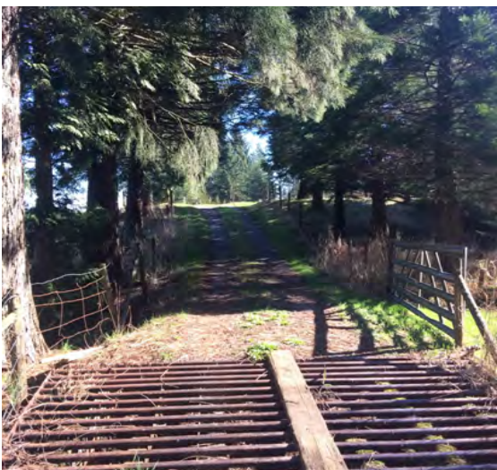
Cattle Bridge at E Creek Culvert
