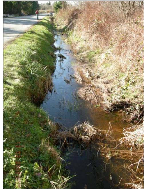
Photograph 16 – 20 th Avenue ditch receives significant flows and drains west to a Class A tributary of Fergus Creek.
