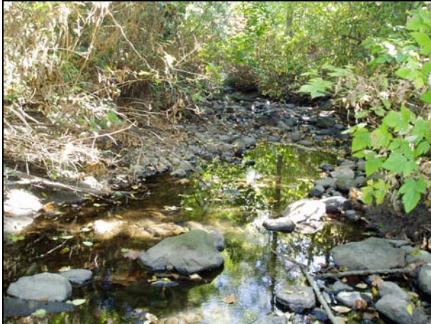
Photograph 7 – Downstream view of degraded channel below 14 th Avenue stormwater connections. Substrate dominated by boulder material and clay with “pock marked” clay surfaces indicating scour and transport of smaller cobble and boulder material -
