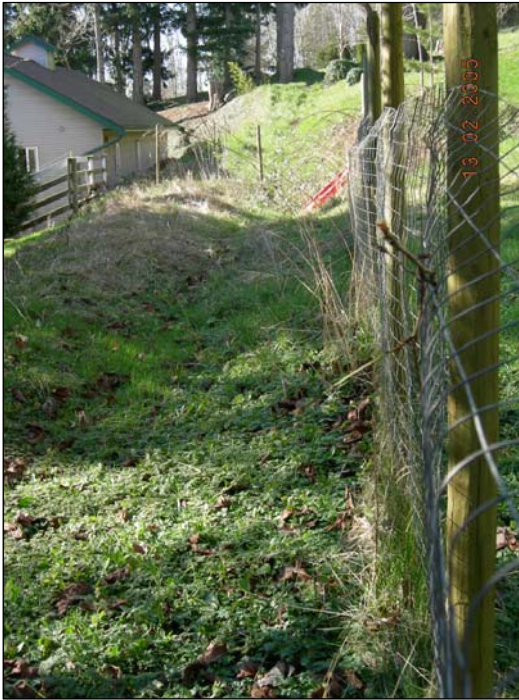
Photograph 23 – Class C swale located above residential property located at 16733 16 th Avenue.
