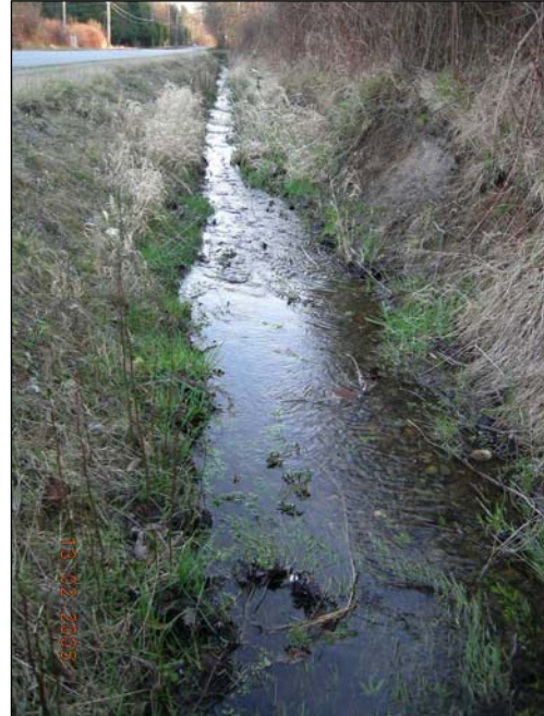
Photograph 18 – Downstream view of 164 th Street west ditch with alluvial substrate, visible scour and sustained flows.
