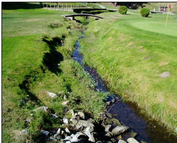
Photograph 10 – Upstream view of modified channel through Reach 3. Visible bank slumping suggests initial channel widening.
