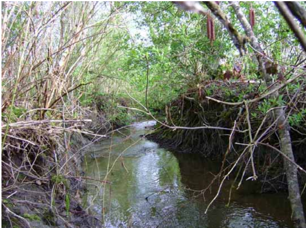
Photo 8: Channel erosion is evident in EC-3.
