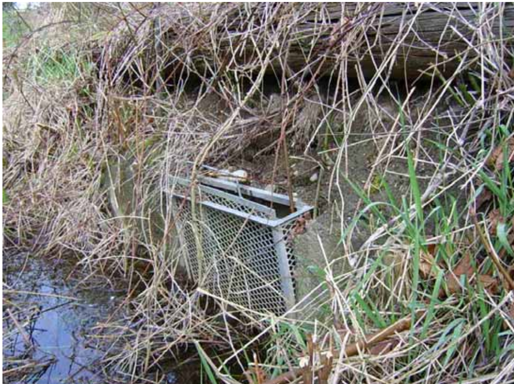
Photo 10: Metal grates cover most culverts under a small access road at EC-4. Open culverts are only accessible during high flows.
