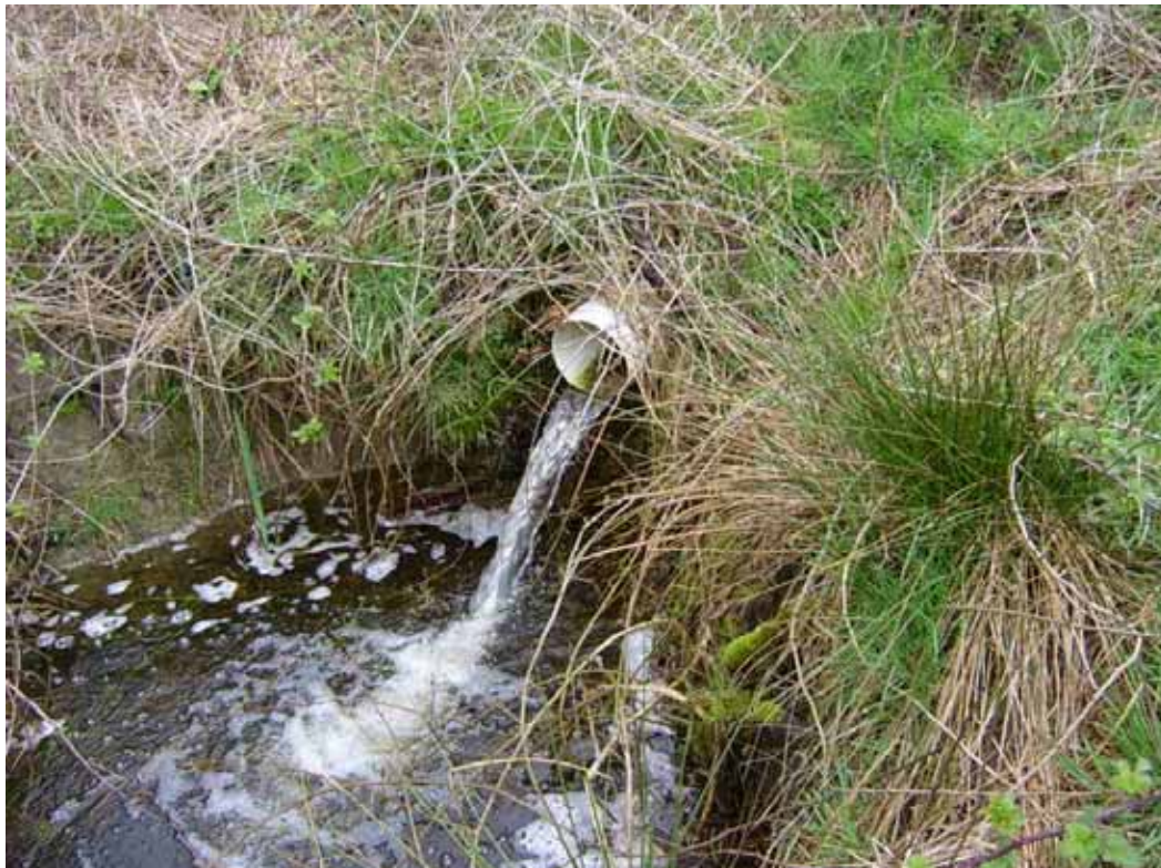
Photo 25: Vandrishe Brook VB-1 has a barrier at the inlet of the lower pond.
