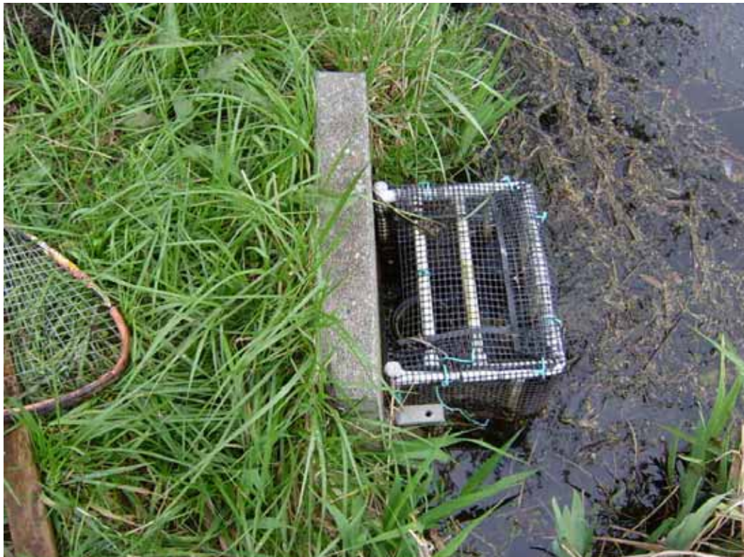
Photo 27: Outlets of third pond in VB-1 are barriers to salmonid migration.
