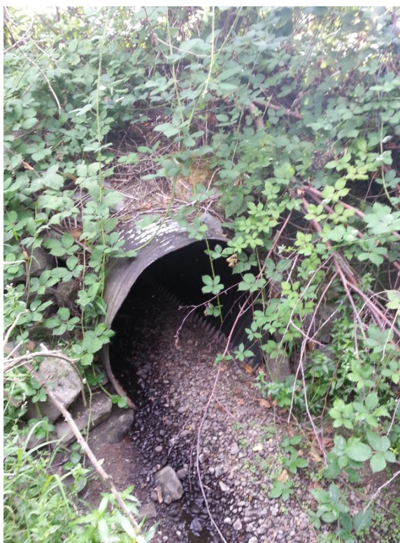
Photo R Downstream End of Hwy 99 Culvert
