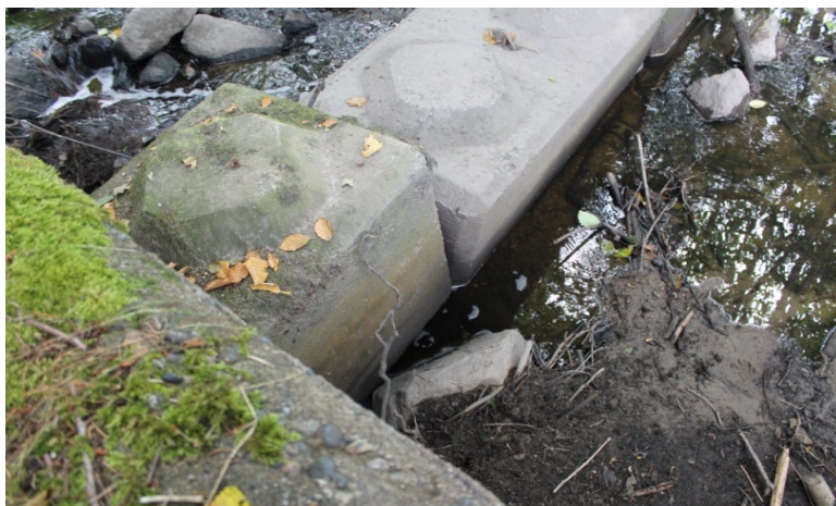
Photo Q Existing Lock Block Weir
