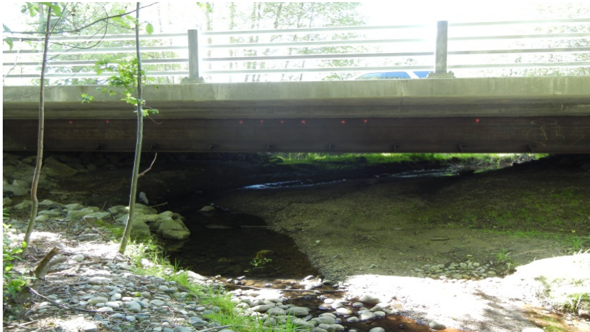
Photo L Downstream of 34 Ave. Bridge
