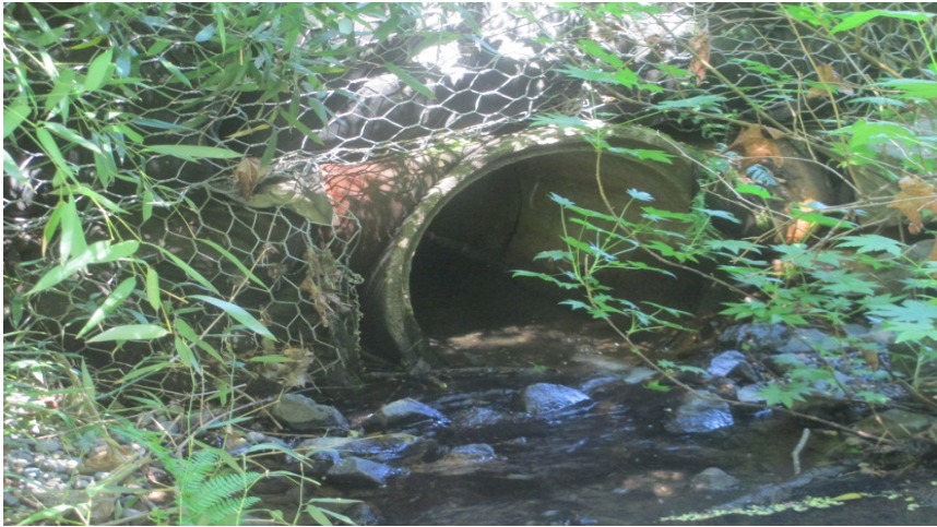
Photo J Culvert Crossing at Winter Crescent
