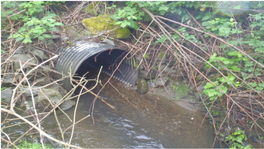
Photo O Downstream of Highway 99 Culvert
