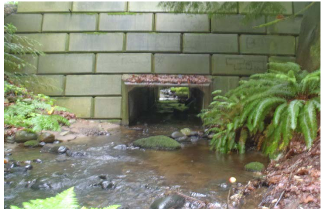
Photo F Upstream of Box Culvert
