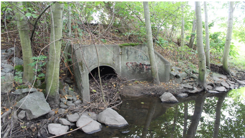
Photo P Upstream of Highway 99 Culvert
