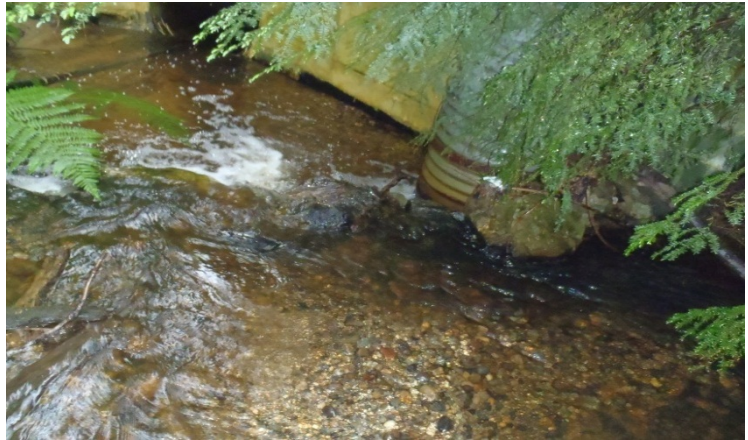
Photo B Riffle Upstream of Crescent Road Culvert
