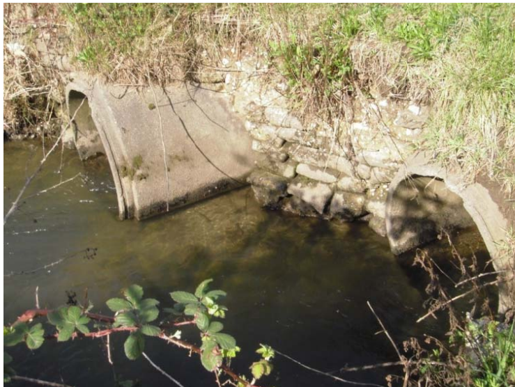
Figure A.7: outlet of McLellan Creek south of Langley Bypass
