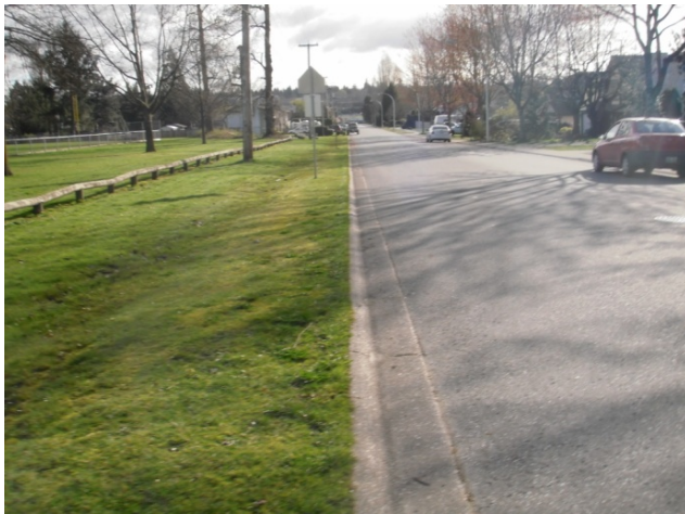
Figure A.13: Shallow Grassed Swale along the North Side of 61A
