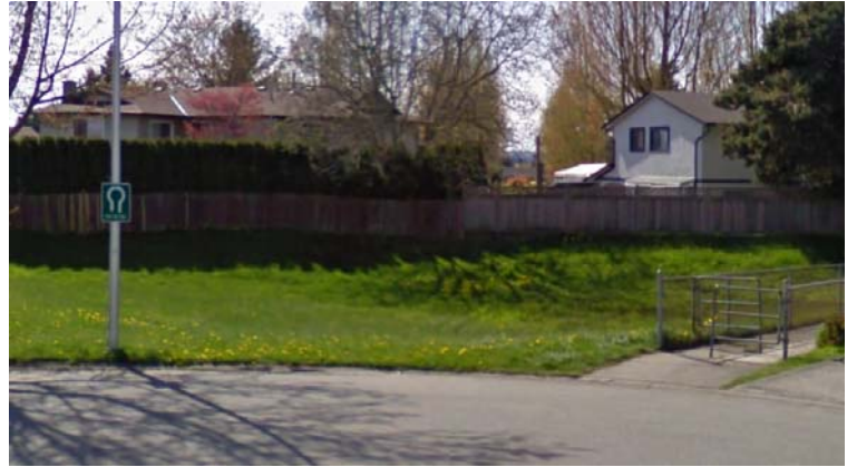
Figure 2.6: Photo F - Dry pond at 58B cul-de-sac
