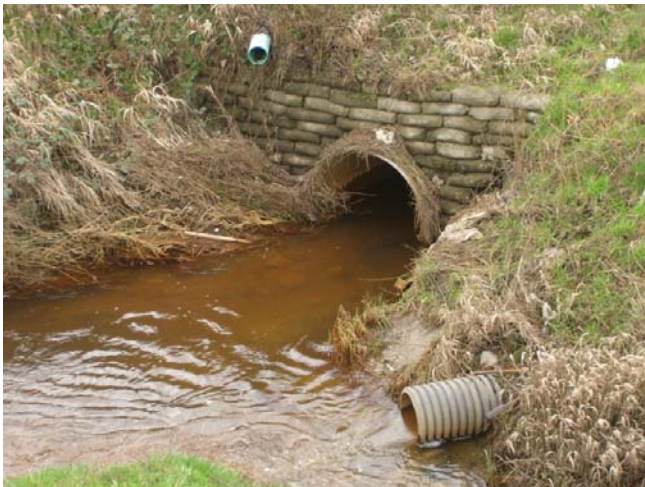
Photo 3: 900mm CMP culvert across 56 Avenue on the east side of 168 St.
