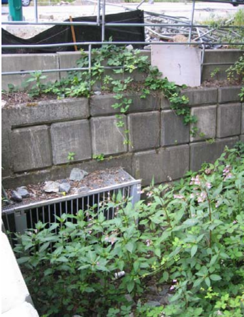
Photo 1: 1800mm Ellipse culvert with gate corner 64 e Avenue and 194 e St.
