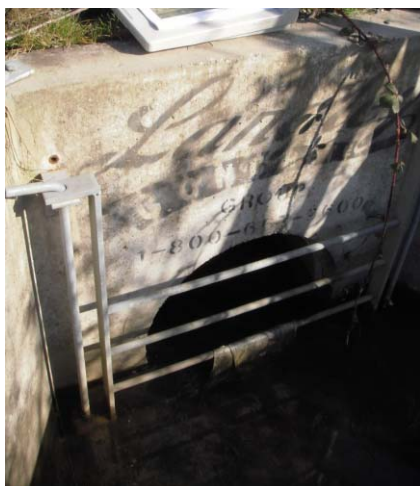
Figure A.2: Outlet of storm sewer system
