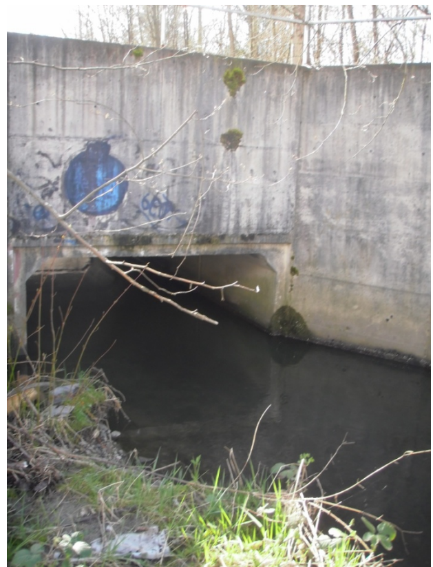
Figure A.10: Box Culvert on lower McLellan Creek.
