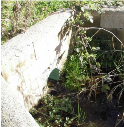
Figure 2.2: Photo B-Storm outlet a 54 th Ave
