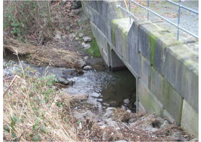
Photo 2: 1200mm x 3600m box culvert across 57 Avenue
