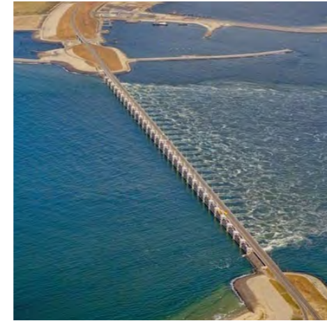
Openings in dam, Oosterscheldekering image: http://www.amusingplanet.com/2014/04/the-netherlands-impressive-storm-surge.html
