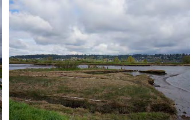
Land eroding outside dyke
