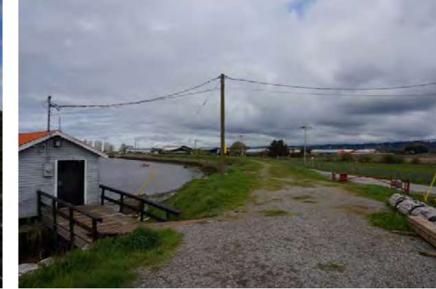
Dyke structure agricultural land
