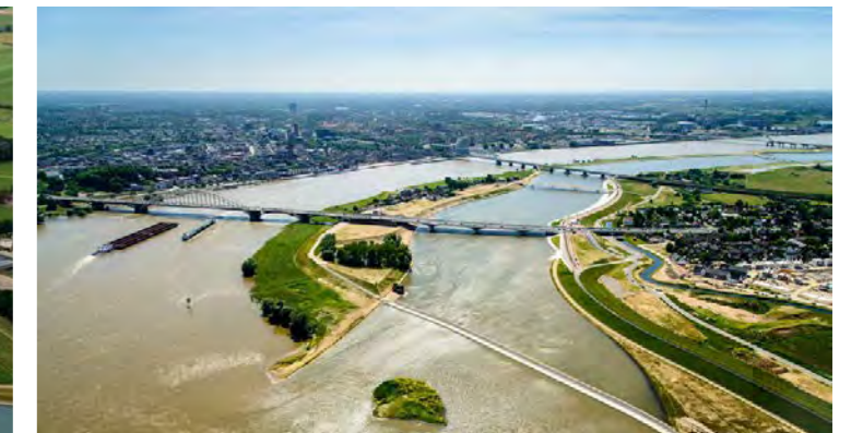
Room for the River, Nijmegen, NL
