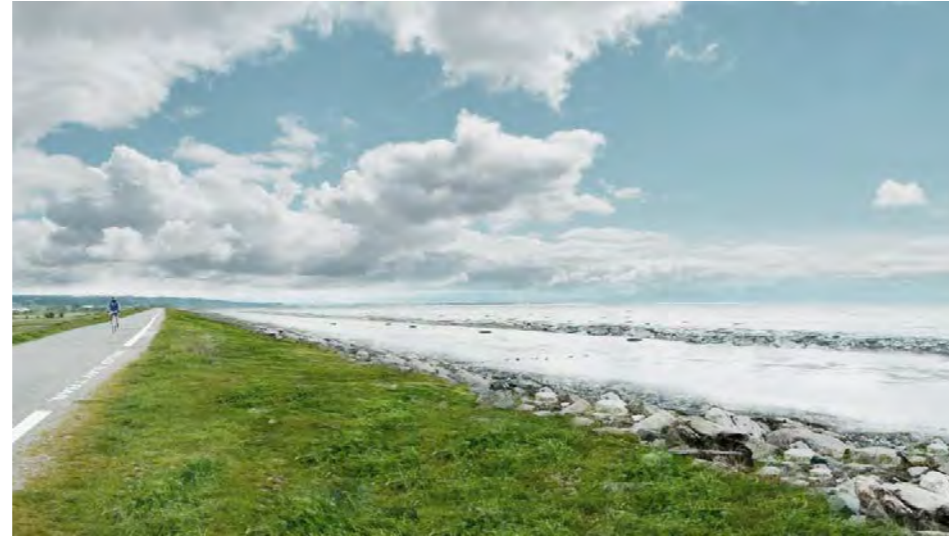
Step 1: Dyke raising in combination with a green slope, a protective dam, and recreational path
