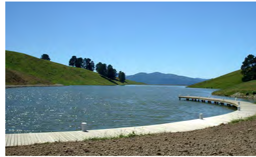
FRESHWATER PONDS: IRRIGATION WATER STORAGE, MARLBOROUGH, NEW ZEALAND HTTPS://TEARA.GOVT.NZ/EN/PHOTOGRAPH/19609/DAM-WATER-STORAGE
