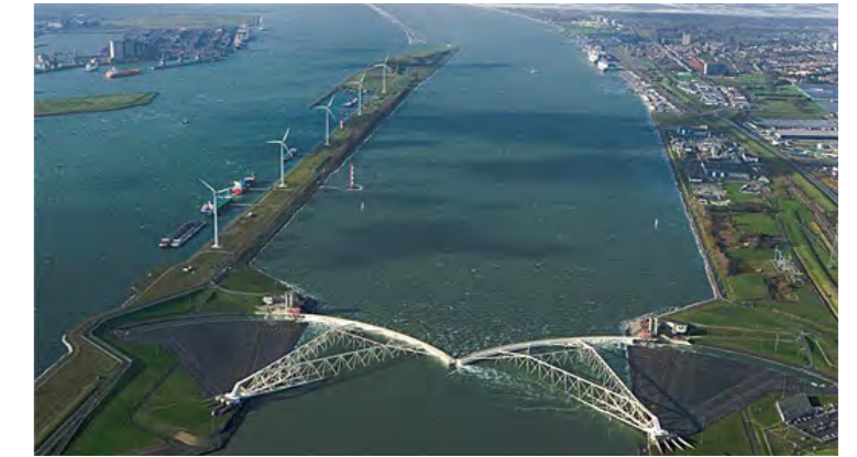
Maeslantkering, Rotterdam, NL image: https://s-media-cache-ak0.pinimg.com/236x/e8/15/07/e8150762ae3457b0ecbedfd96b0f581.jpg
