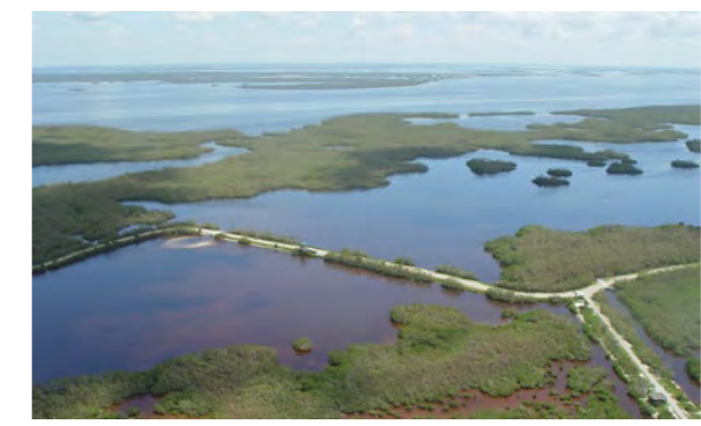
Raised road structures image: http://refugeassociation.org/wp-content/uploads/2014/03/ding.jpg
