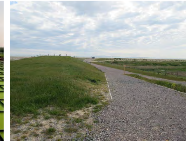
Managed realignment, Medmerry, Sussex, UK
