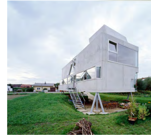
House on stilts
