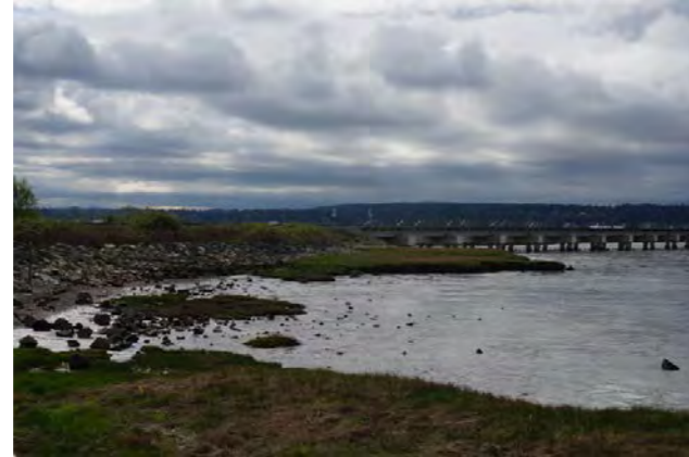
Dyke + BNSF Railway bridge
