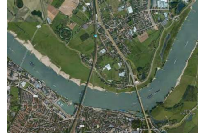
Relocation of small town, Lent, for Room for the River project in Nijmegen (Before) image: http://citiscopes.org/story/2015/dutch-city-makes-room-its-river-and-new-identity
