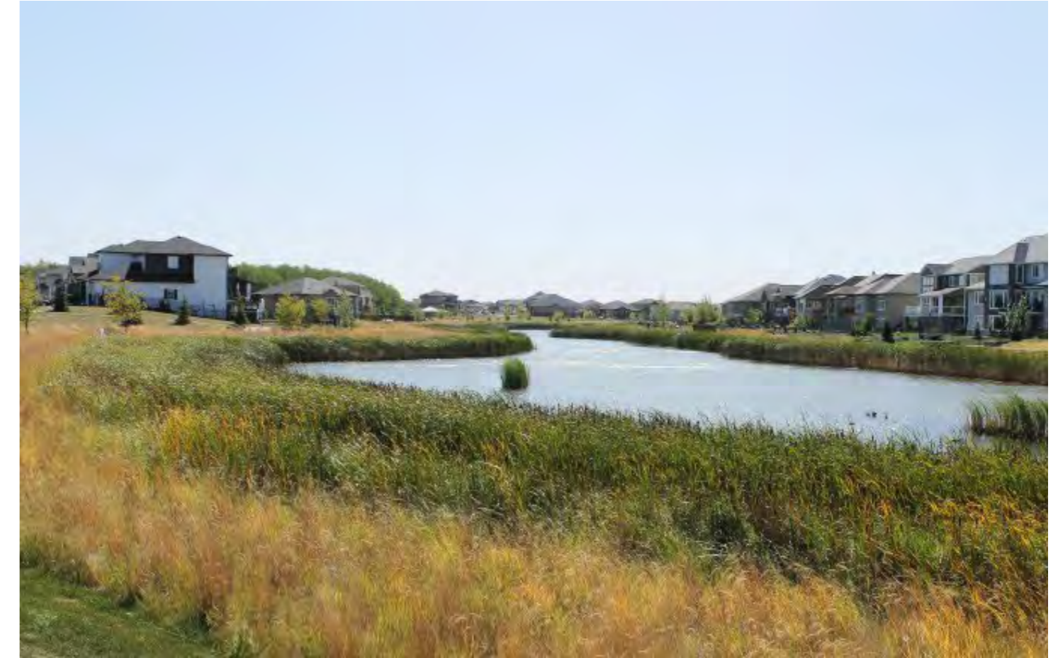
Channel flooded during peak flow.
