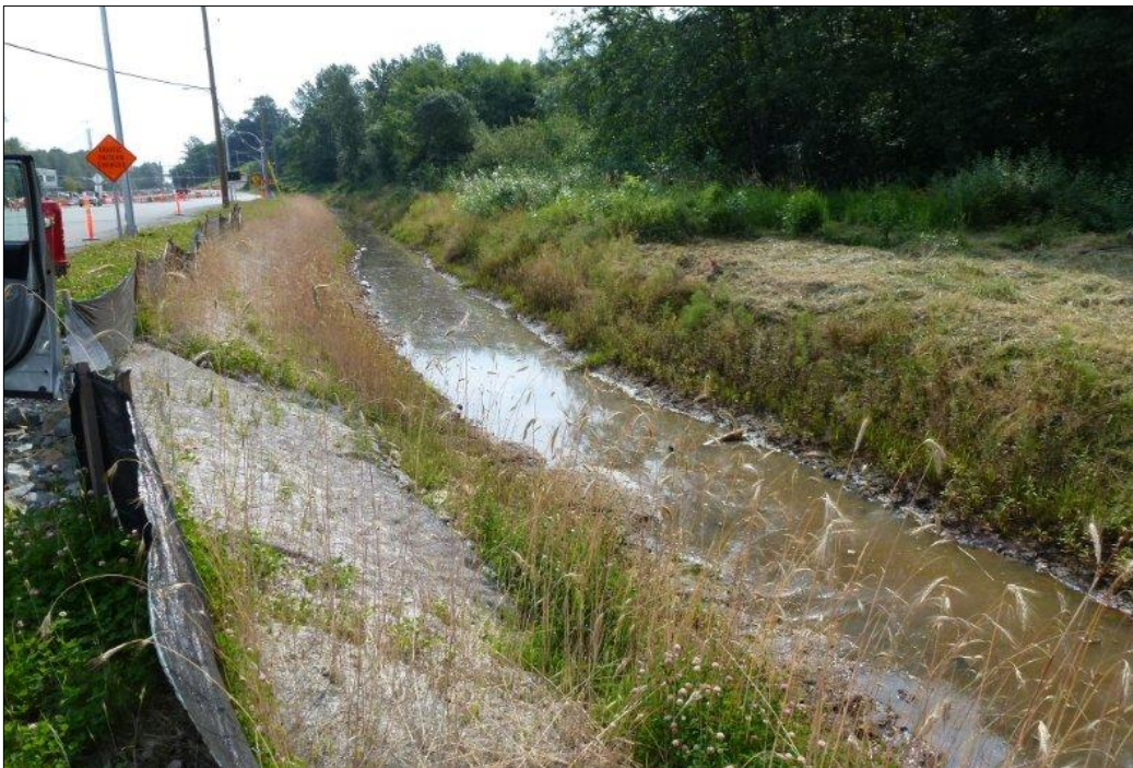
Photo 7: Southward Creek at large constructed channel south of 116 th Ave. & SFPR.
