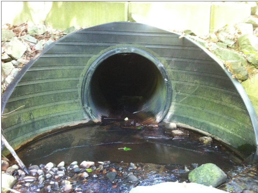
Photo 2: Bolivar Creek fishway at 112 Ave. looking downstream (North).
