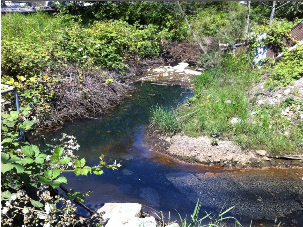
Photo 6: Large constructed channel south of 116 Ave. & SFPR at 136 St looking East
