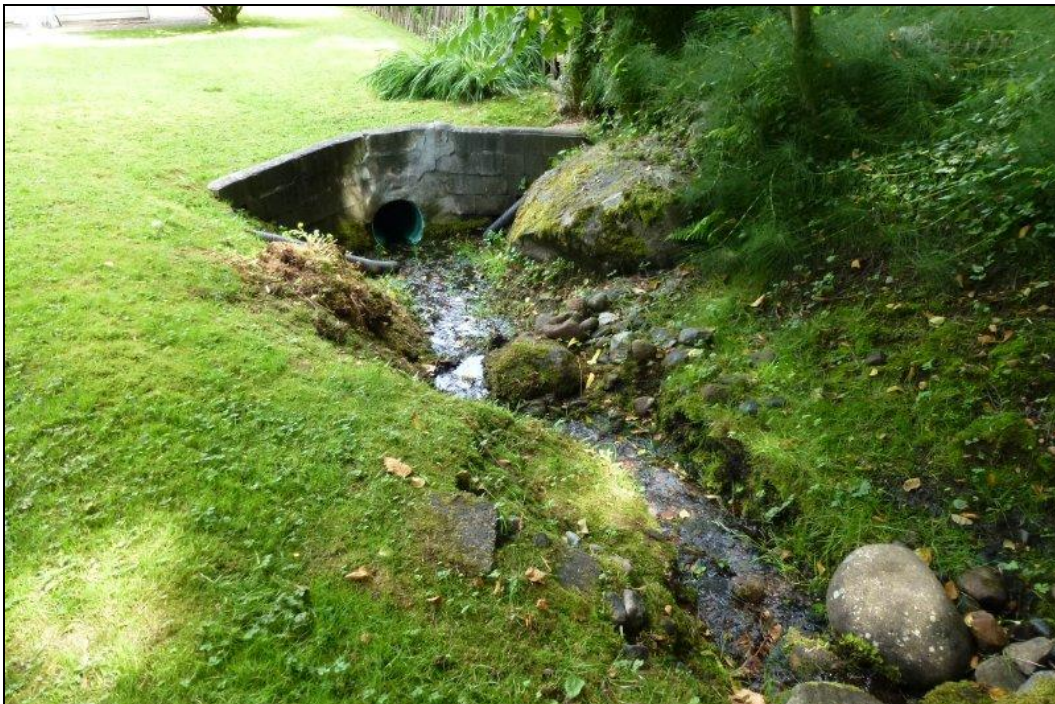
Photo 14: Dingwall Creek at culvert inlet beneath 14026 – 116 Ave. residence & 116 Ave.
