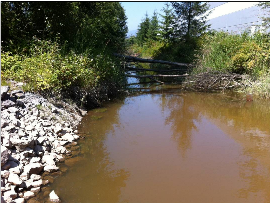
Page 9: Infilled channel/ fish migration barrier, 116A Ave. & 130 St. looking West
