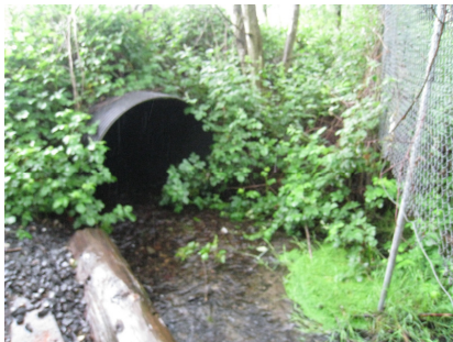
Watershed R1 (culvert inlet)
