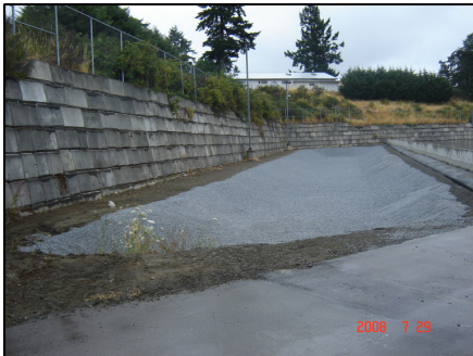
Surface Infiltration Swale
