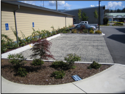
Reinforced Clean Crushed Gravel
