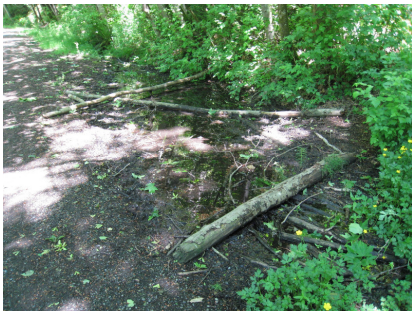
Lower Trail Ditch
