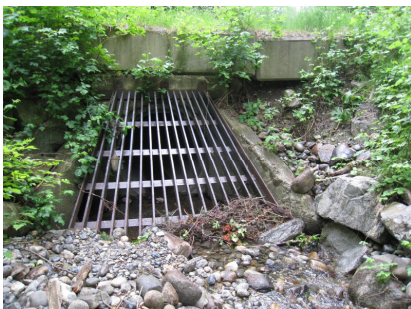
Shaw R4 (culvert inlet)
