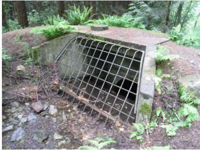
Briarwood R2 (culvert inlet)
