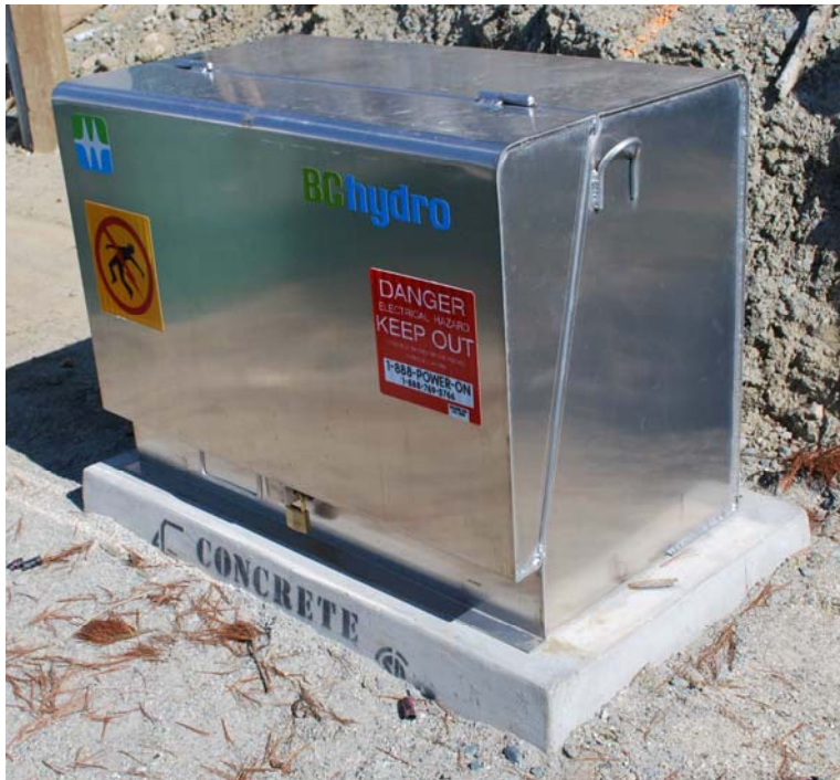
Figure 1: 400 A 120/240 V Service Isolation Kiosk for U/G Service Connection
