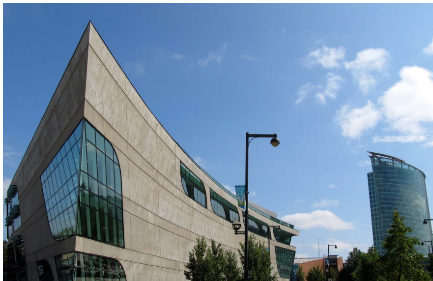
View of City Centre Library
