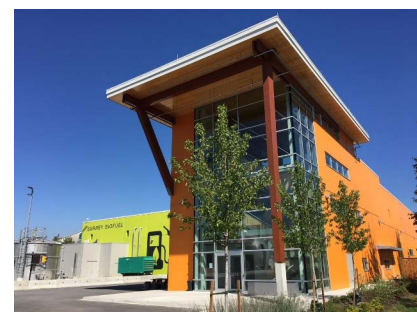
Surrey Biofuel Facility, City of Surrey
