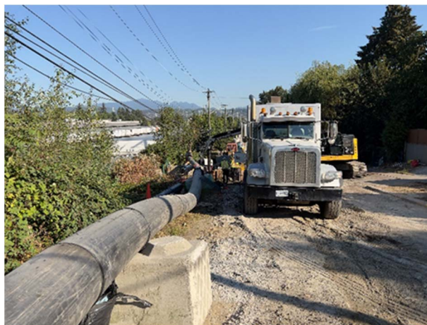
Trunk Sewer Construction on 132nd Street
