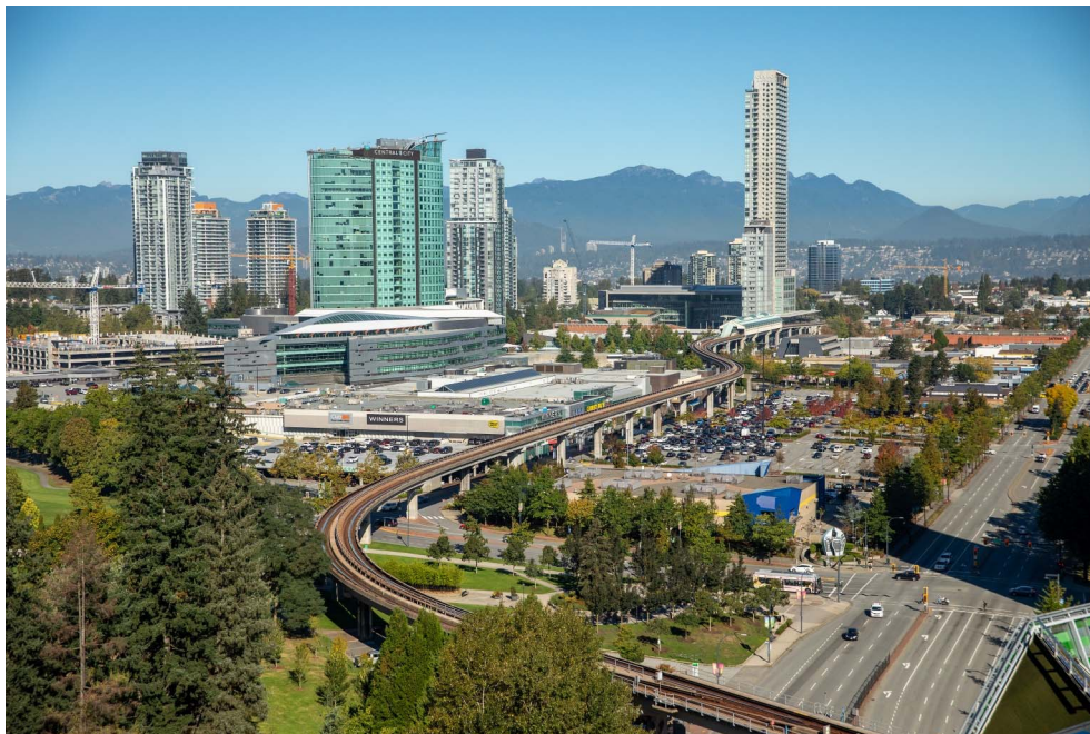
Skytrain track in City Centre
