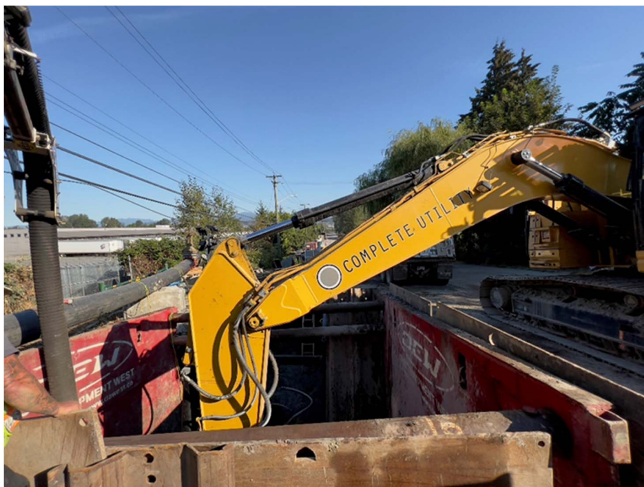
Trunk Sewer Construction on 132nd Street near 114 Avenue
