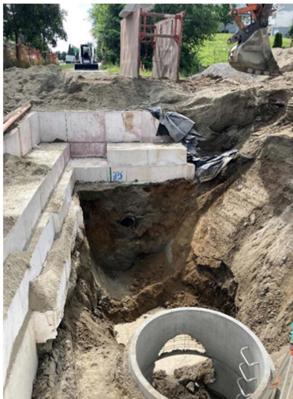
Construction of North Cloverdale Trunk Sewer
