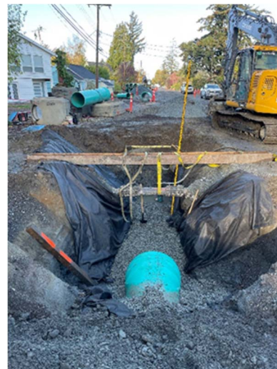
Storm Sewer Construction in Crescent Beach
