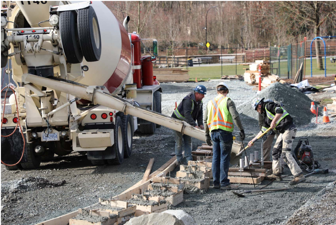
Construction at Hawthorne Rotary Park
