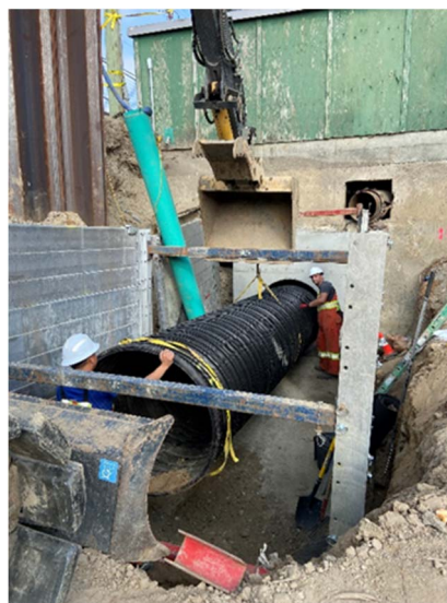
Construction work related to drainage in the City of Surrey
