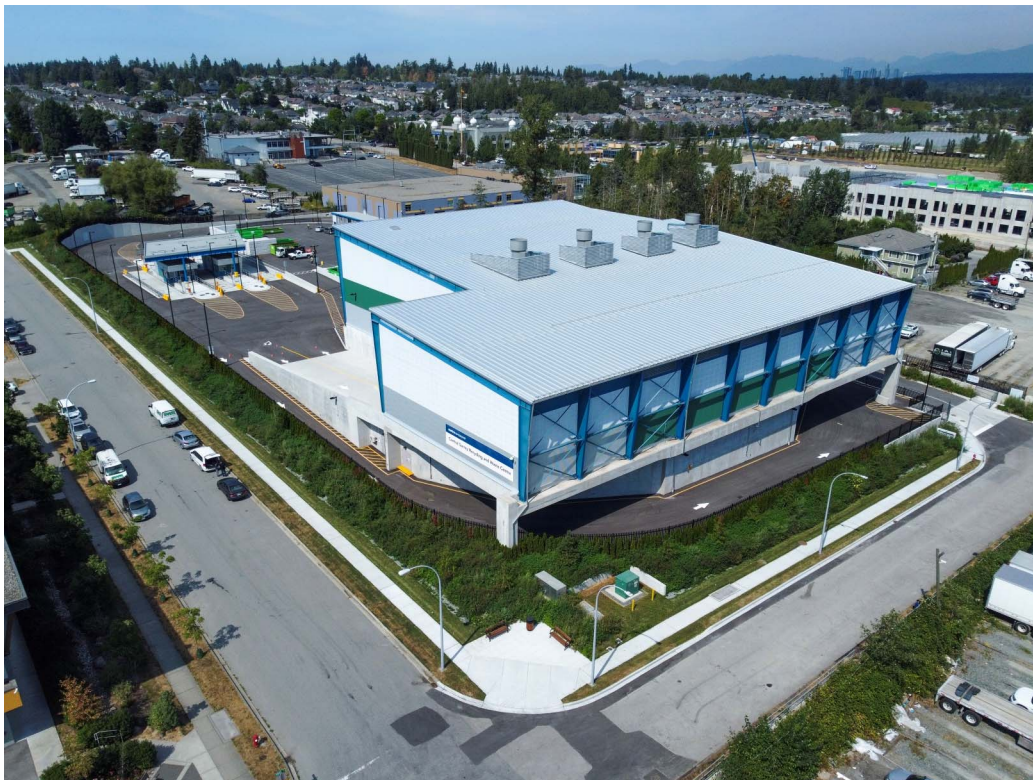
Exterior of Central Surrey Recycling and Waste Centre
