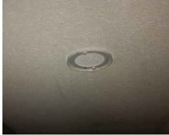
Removed Smoke Alarm
